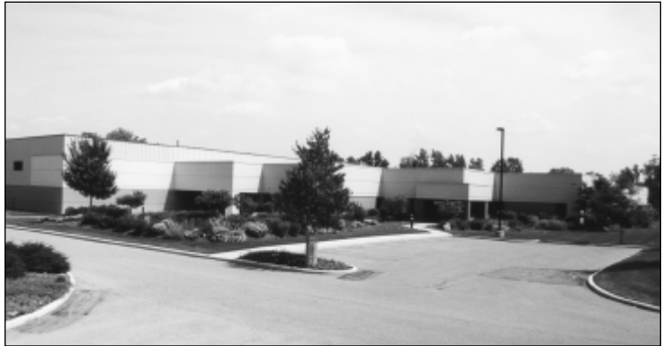
Honeywell's facility in Columbus, Ohio
